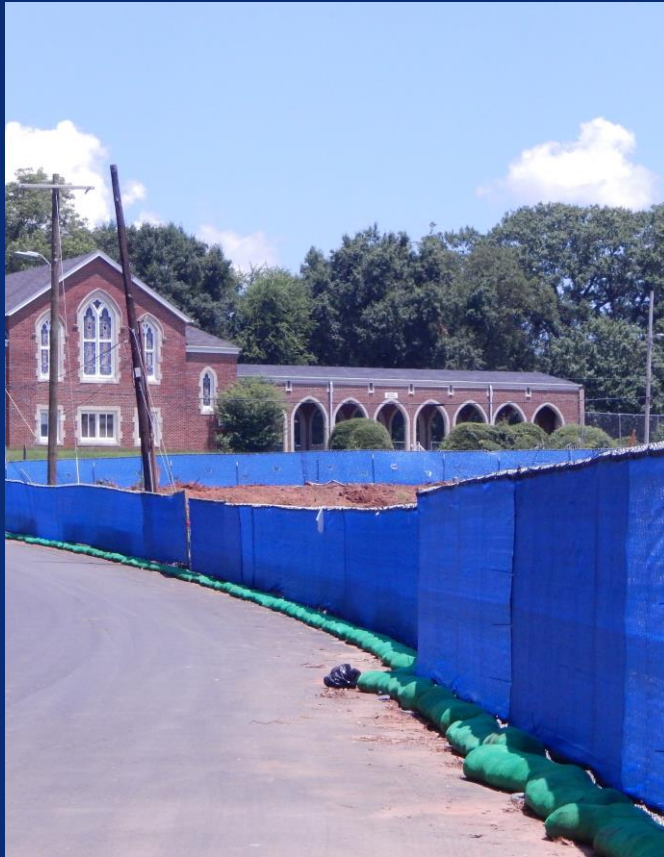
Wind Screen & Erosion Control Installation at South Alvarado
