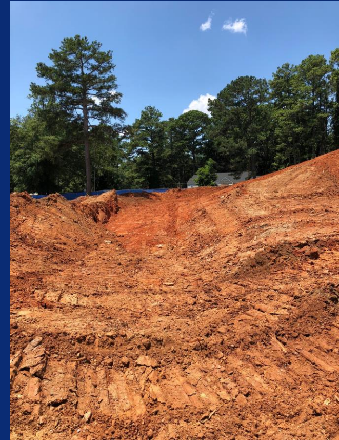
West Side Underground Detention System Excavation
